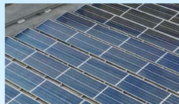
Instalasi Panel Surya Solar Panels Installation
