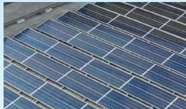
Instalasi Panel Surya Solar Panels Installation
